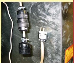
was installed on the other cut end and a mini-extension-cord was made so the original "hard wired" power connection could be restored.) Worked perfectly - a few hours later the indoor temperatures were back to livable ranges.
