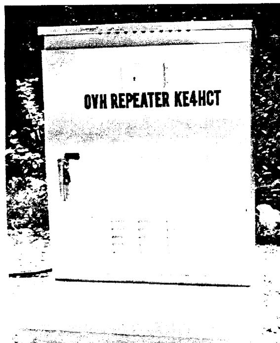
The Finished Tower Box housing the OVH 440 Repeater
